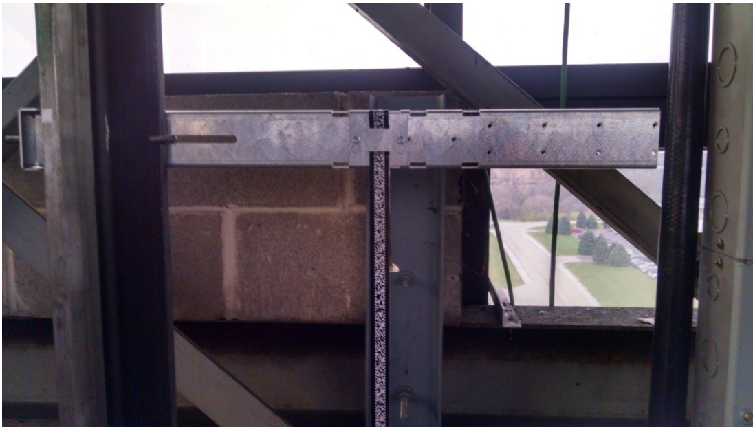
Figure 2.12: Encoded Tape Mounting
