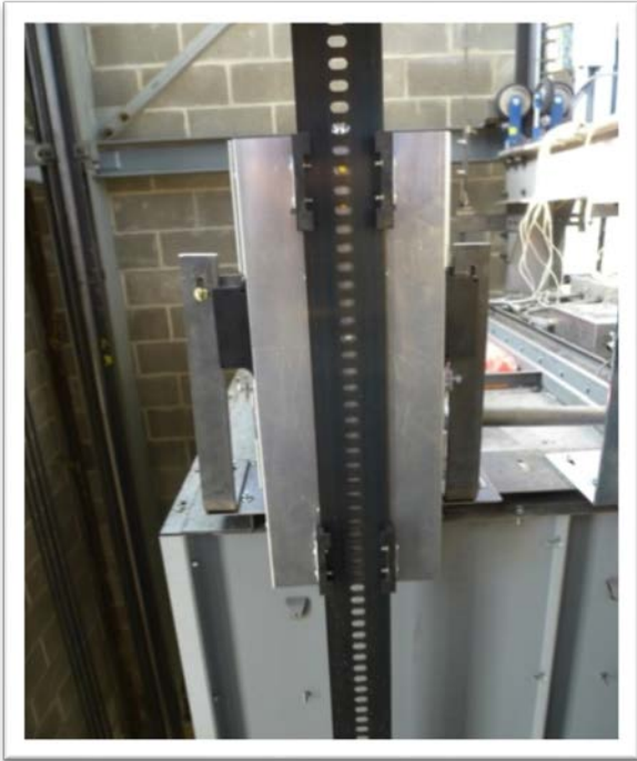
Figure 2.3: Typical Selector Installation
